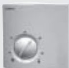
RAA20 speed controller in the front cover of the controller (the controller is located in the space under the curtain)
