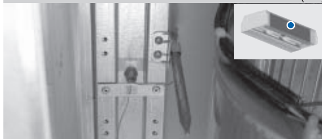
RAA30 speed controller in the front cover of the controller + possibility of switching off the heating (the controller is located in the space under the curtain)
